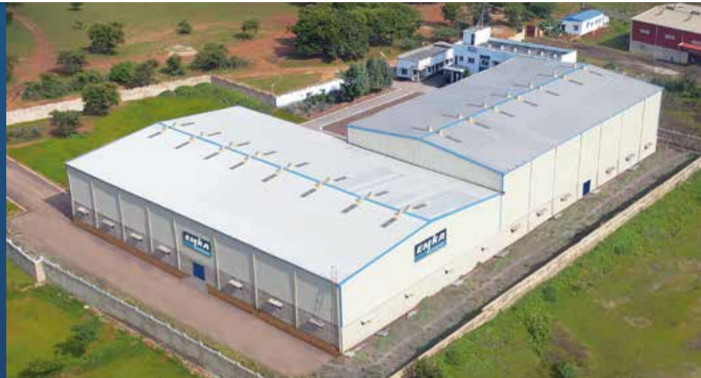
The total covered area is 6,000 m 2 . A state-of-the-art powder coating machine was recently put into operation.
